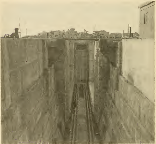
LOCK GATE TRACKWAY AT CHARLES RIVER DAM WHICH WAS FILLED WITH SAND TO LEVEL OF LOCK FLOOR.
